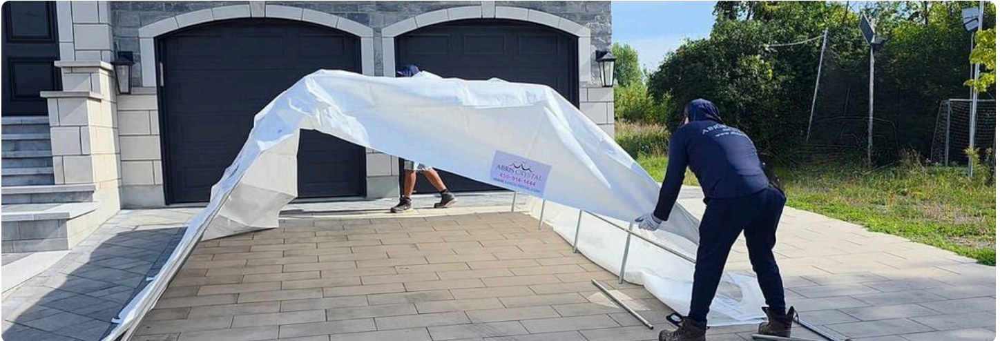
La toile passe par-dessus la structure / The tarp goes over the frame
