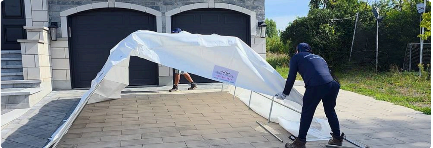
La toile passe par-dessus la structure / The tarp goes over the frame
