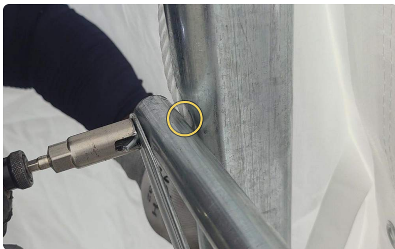
Top corner: the rope locked under the spacer
