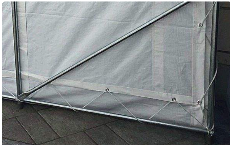
Result: the rope zigzags, nice and tight
