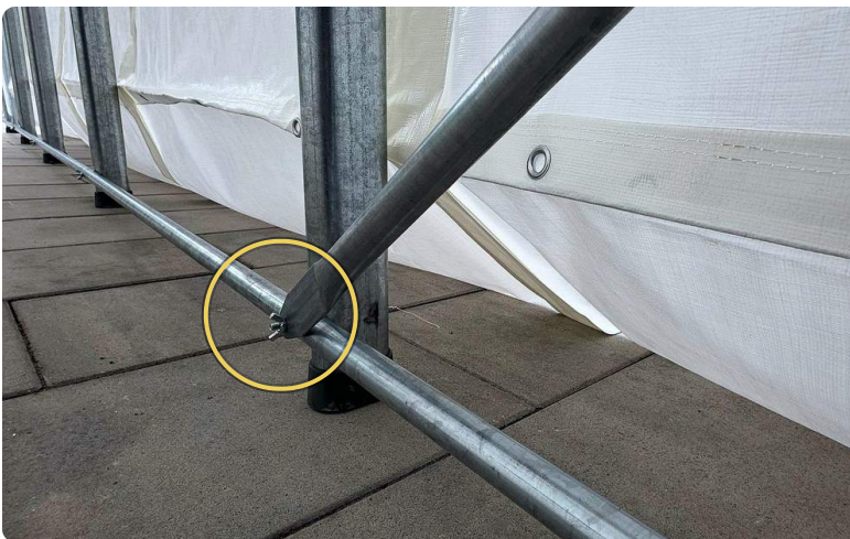
Bottom of the diagonal brace: same B2 bolt as the spacer
