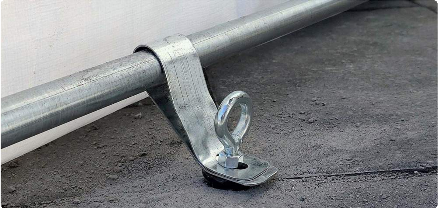
On pavers: permanent anchor (photo: single shelter)
