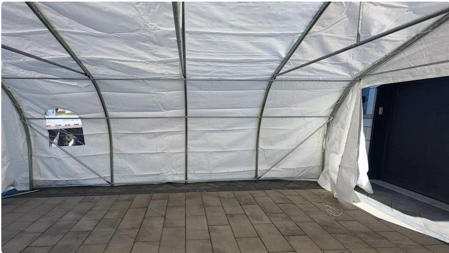
One side from inside: legs in line, a diagonal brace at each end
