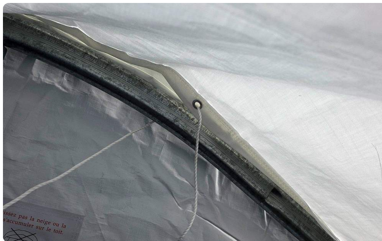
Seen from inside: the velcro and the rope
