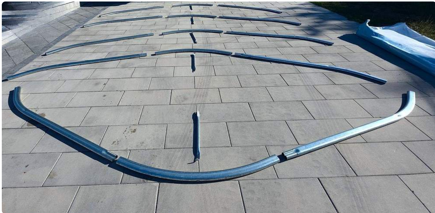
One arch, without its door bar: 2 corners, centre, T-bar
